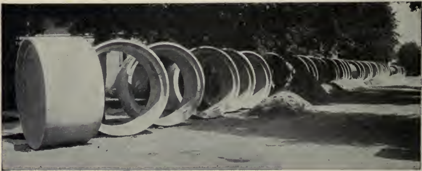
84-INCH CONCRETE PIPE READY FOR INSTALLATION AT KOKOMO, IND. Kokomo's first 24-inch concrete sewer pipe was laid in 1873 and is still in service
